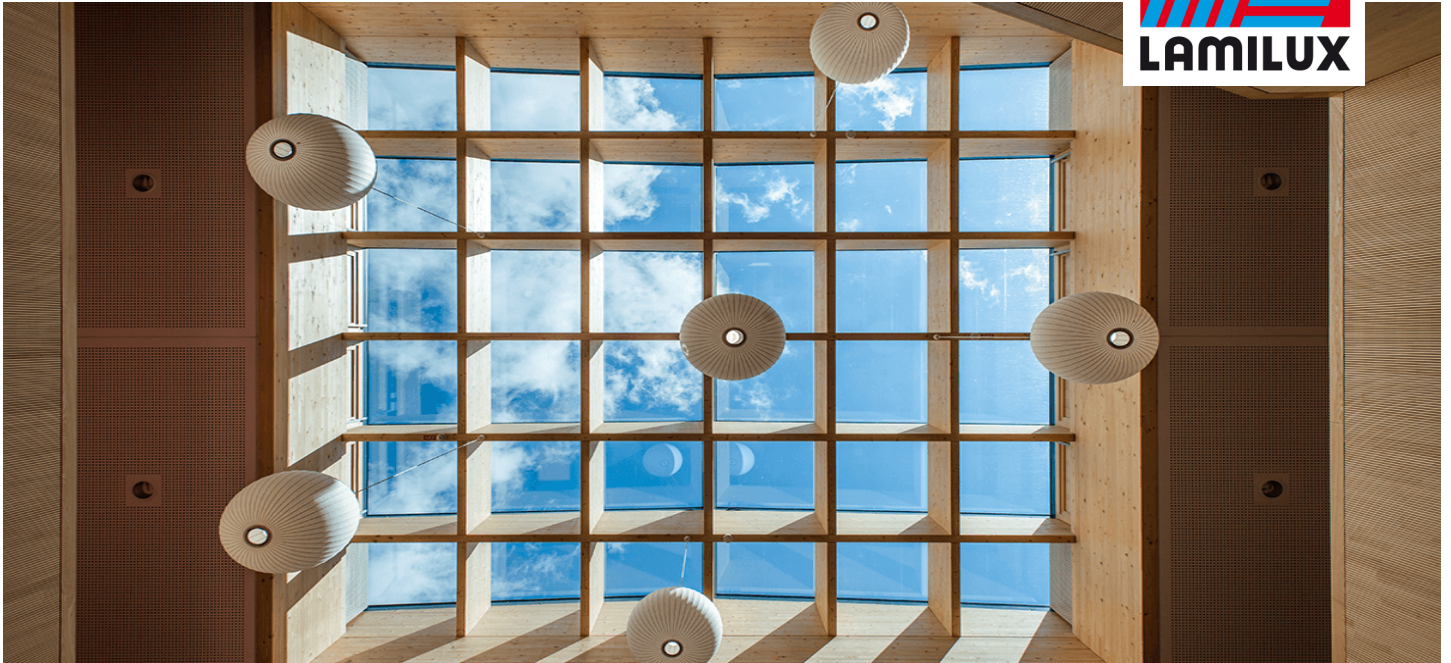
Day Care Centre, Frankfurt
