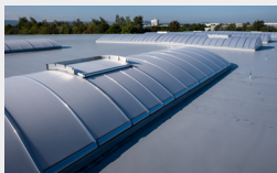
CONTINUOUS ROOFLIGHT
